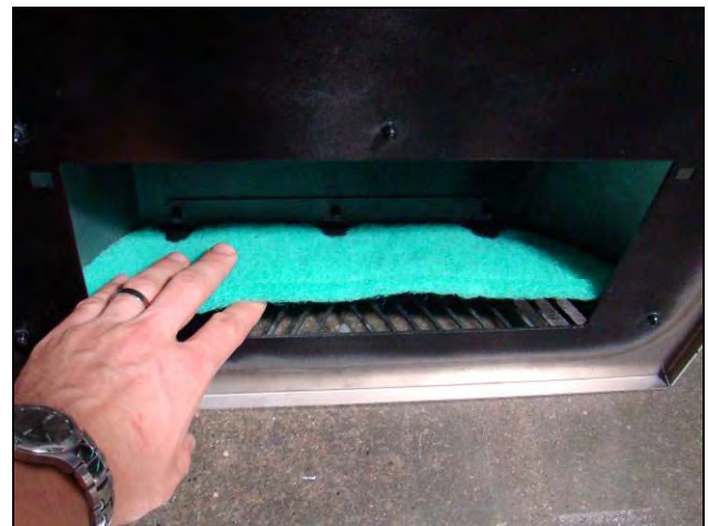
Figure 28: Removing Filter Medium
