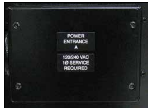
Figure 5: Myers Hub Power Termination Box
