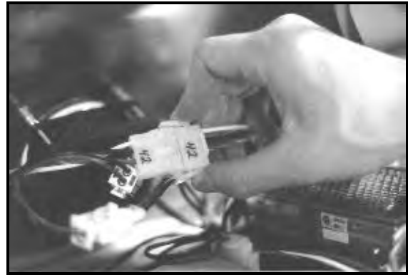
Figure 25: Disconnecting LED Module Panel Power Cable
