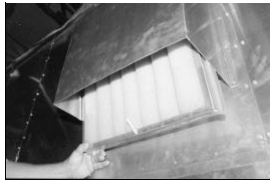
Figure 54: Filter Removal - Rear Access
